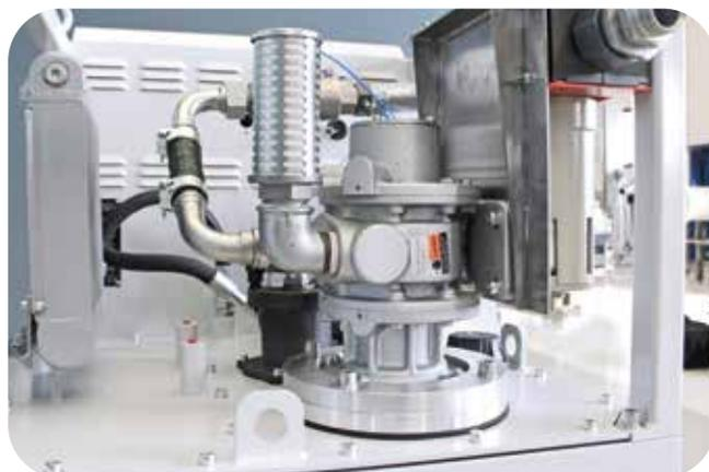
Hydraulic oil filter with mechanical indicator for hydraulic oil filter change warning.
